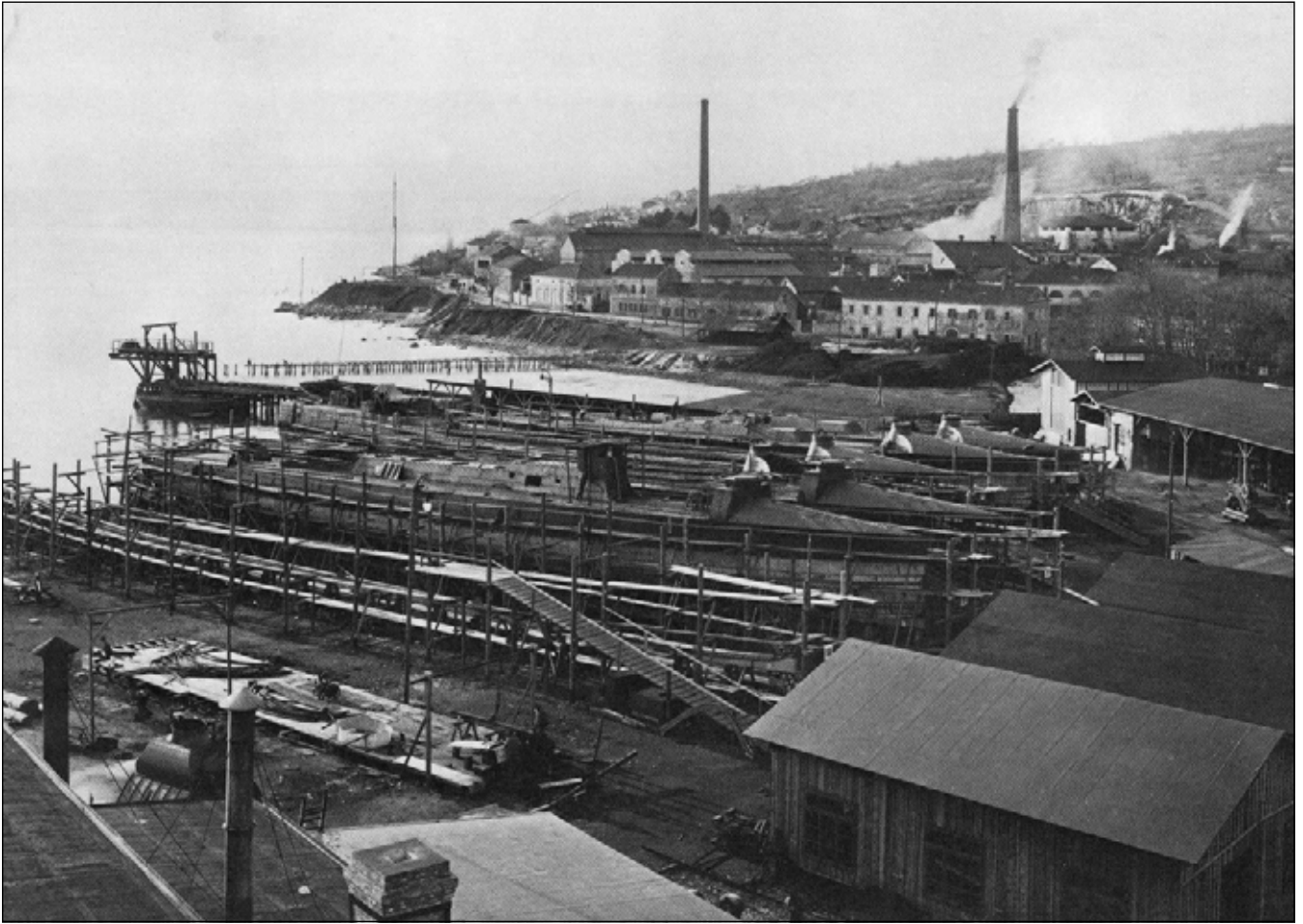
34 The Danubius Shipyard in Fiume-Bergudi with Huszár class destroyers and Kaiman class torpedo boats under construction
