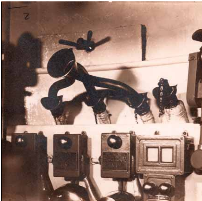
72 Inside one of the fire control positions of the 15 cm/50 battery
